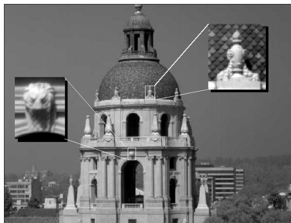
Fig. 8. Image of Pasadena City Hall.
